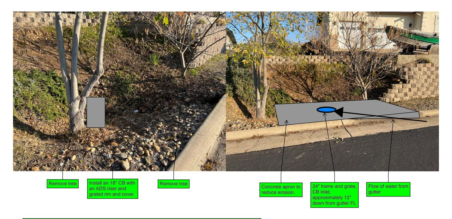
Cost for the removal of the trees, dig out base for CB, pour base and riser, backfill around base, grade and pour apron and grade around the new catch basin.
